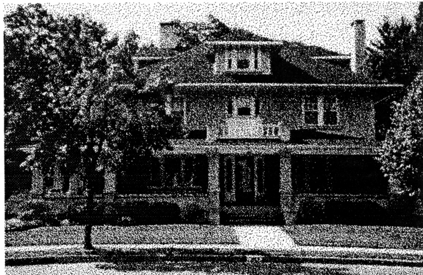
The Charles A. Mason house (1915) located at 408 South Main Street
