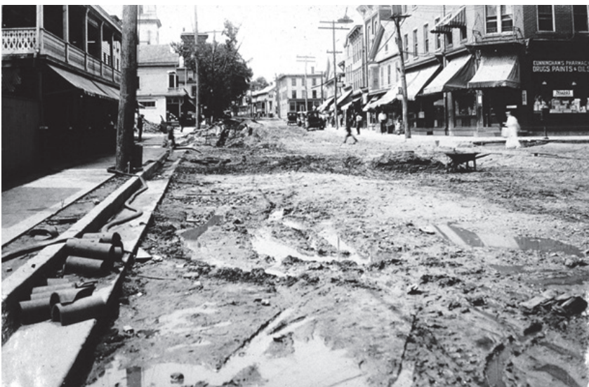
Main Street at the time it was being paved.
