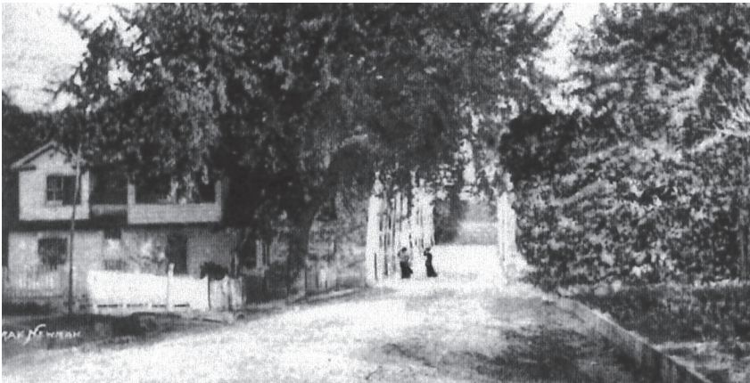
East Ward Street and the Ward Street Bridge
