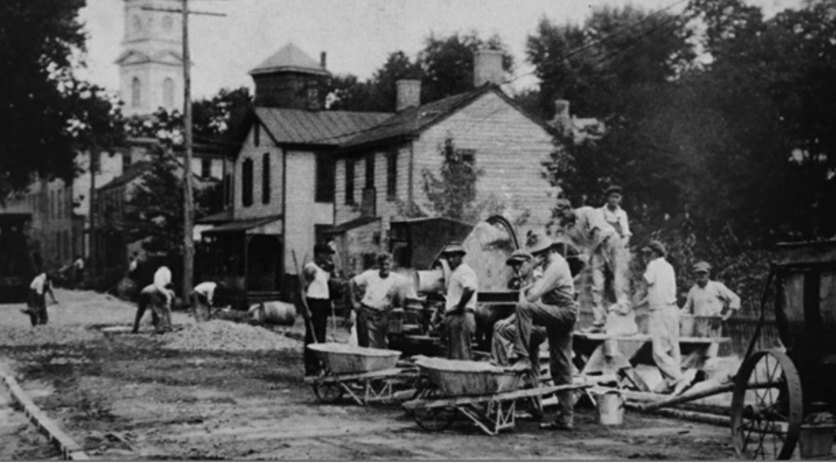
1920 Mercer Street Concrete pouring of State Highway 7, now Route 33
