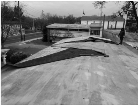
Freight Station Roof
