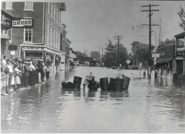
Main Street becomes a public pool during 1934 flood.
