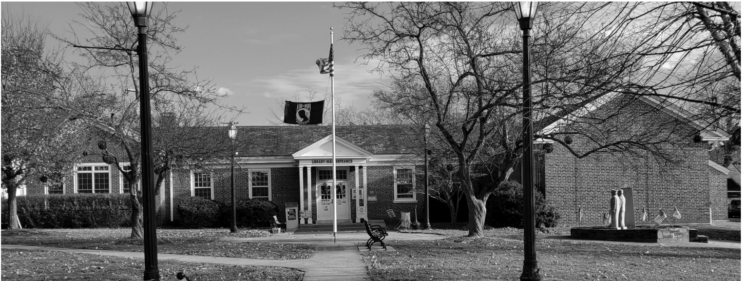
The center section is the original library. The wings were added later.
