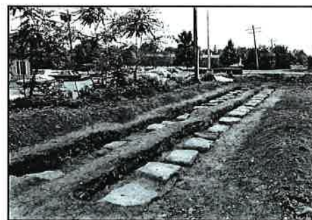
Before wooden ties were used to support rails, large blocks of carved stone, called sleepers, held the rails in place. Sleepers were uncovered in Hightstown because the Camden and Amboy Railroad was only the third railroad built in the United States. Wooden ties were just one of many inventions to follow. HEWHS
