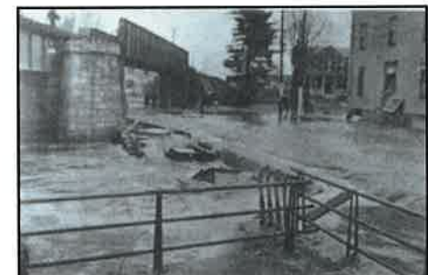
Water pours over the road into Rocky Brook. Notice the old mill on the right.
